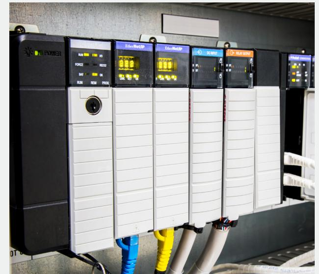
PLCs typically come in two formats – compact and modular. Compact PLCs are a standalone device containing all the necessary devices. Modular PLCs start with a main module, and additional expansion modules can be fitted for more functions, upgrades or larger installations.
